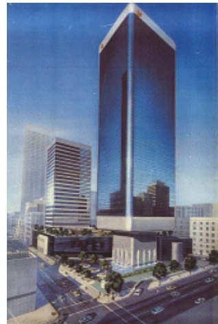
High rise building designed to withstand car bomb effects
